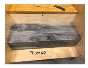
Fitting of preformed LVT "Six Degrees" step down riser treads, shown in Photo #2 and manufactured by Roppe Holding Company, leave you a few options.
